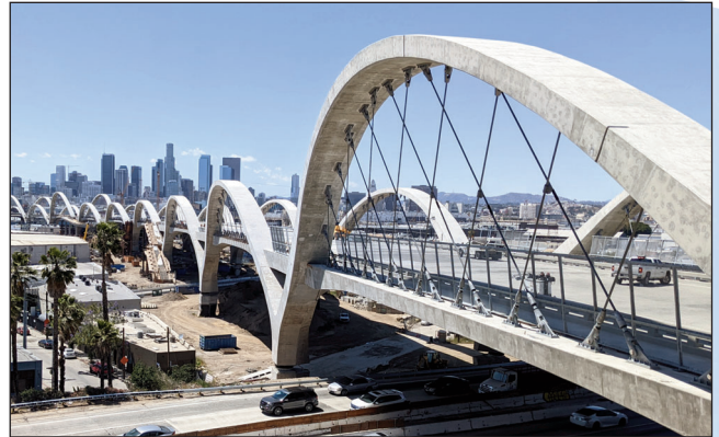
Sixth Street Viaduct, Los Angeles, USA / Kunde/Customer: COWI North America
